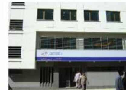
IBC Defence – Post Revamp
